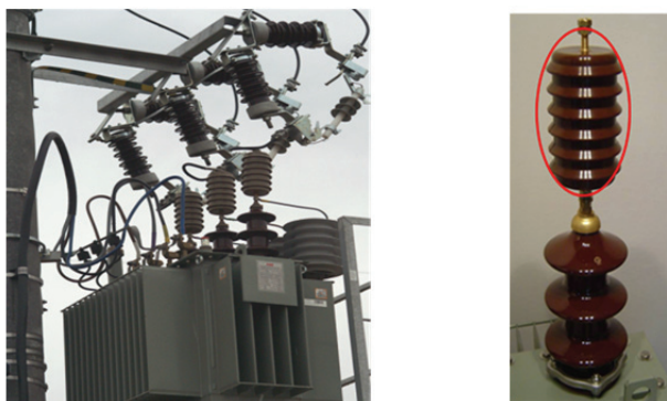
Fig. 16 VFTs suppression device pilot installation
