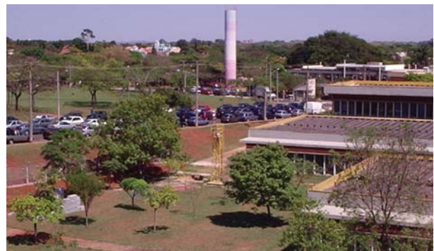
Fig. 5. Microwave link (building top-floor vision).
