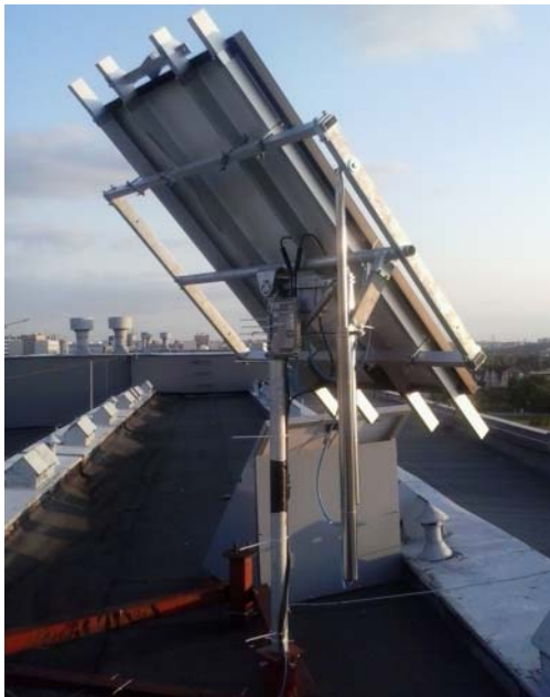
Fig.2. A view of the tracking photovoltaic system installed on the roof of the Poznań University of Technology building
