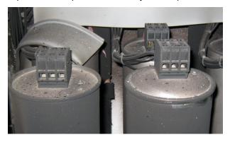
Fig. 10. Photograph of an example capacitor bank step after 5 years of operation
