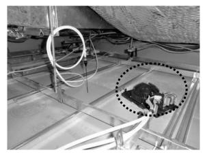
Fig.4. An antenna of a telemetry system (pole-type) and a LED socket (hatched circle) in the ceiling
