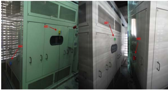
Fig. 4. The location of the signal sensor installation
