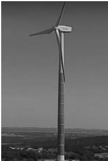
Fig. 4. Wind turbine in Albacete, Spain [3],[21]
