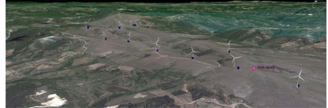
Fig. 7. Organised wind park after optimisation of the turbines position
