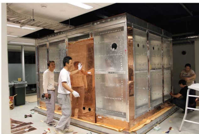
Fig. 5 The assembling of room for MEG diagnostics [9]
